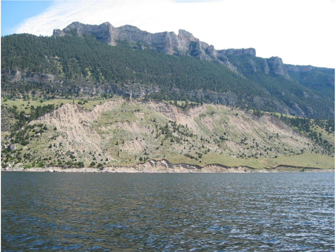
Figure 26 - Bighorn Lake Landslide Area Upstream of Range Line 3A.
