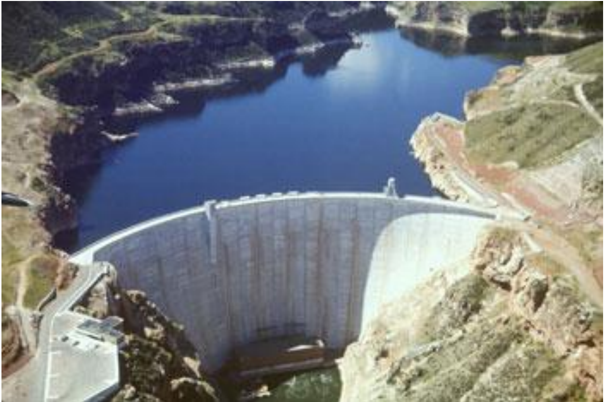
Figure 2 - Downstream Face of Yellowtail Dam.
